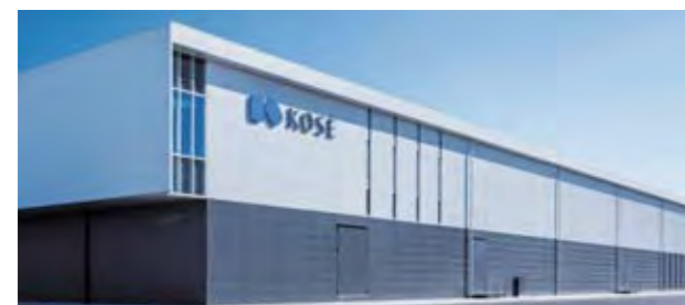
New manufacturing facility at the Gunma Factory
