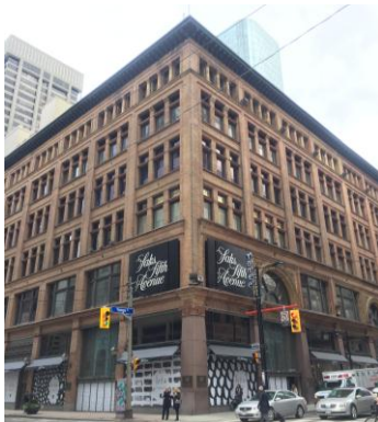
Saks Fifth Avenue, Eaton Centre store
